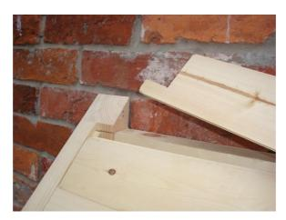
8. Fix the small wooden wedge level with the end of the rafter. The fascia board can now be fitted level with the top of this wedge.
