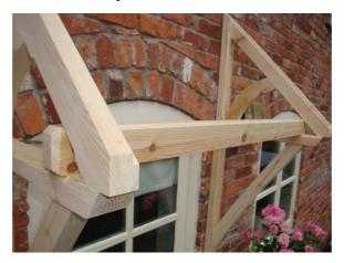
5. Drill and fix with screws, the centre rafter/s.
