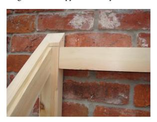
4. Fix the front wall plate into position with screws. It should be project either side of the side brackets by 10mm.
